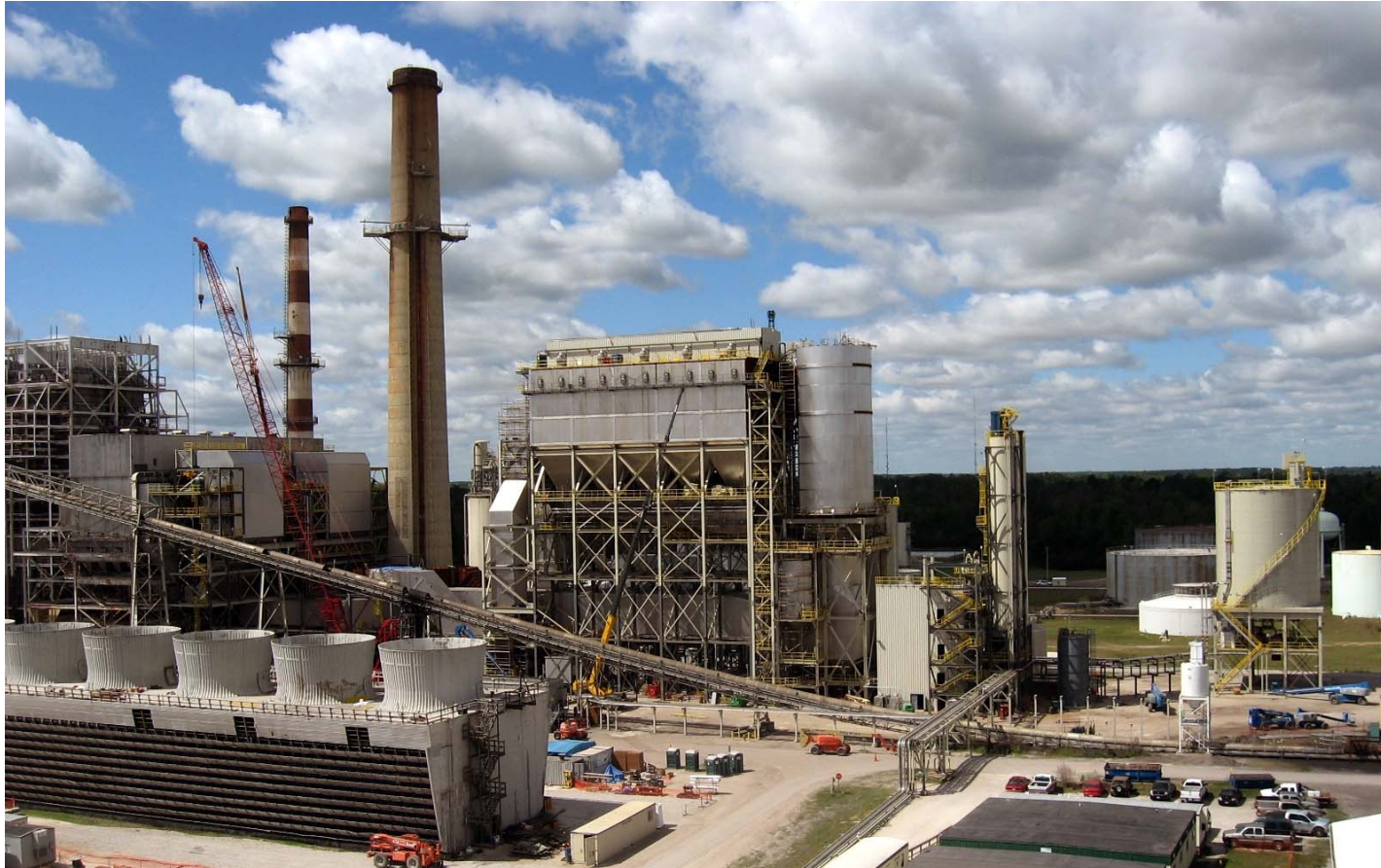
Photo Courtesy of Gainesville Regional Utilities
